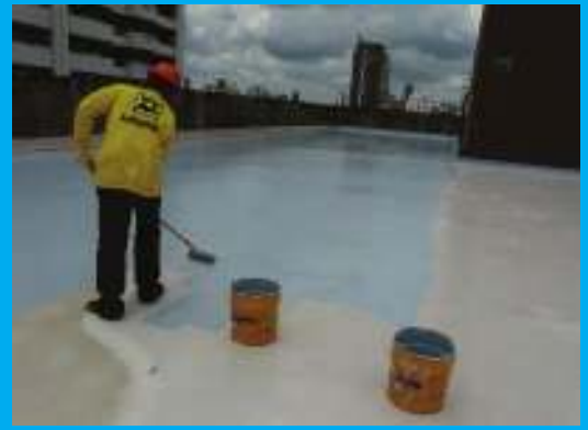
Roof deck waterproofing system
