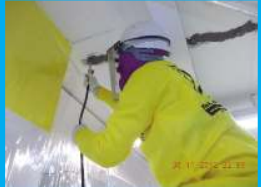
Epoxy injection to crack
