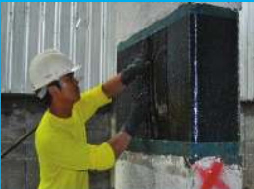
Carbon fiber wrapping to column
