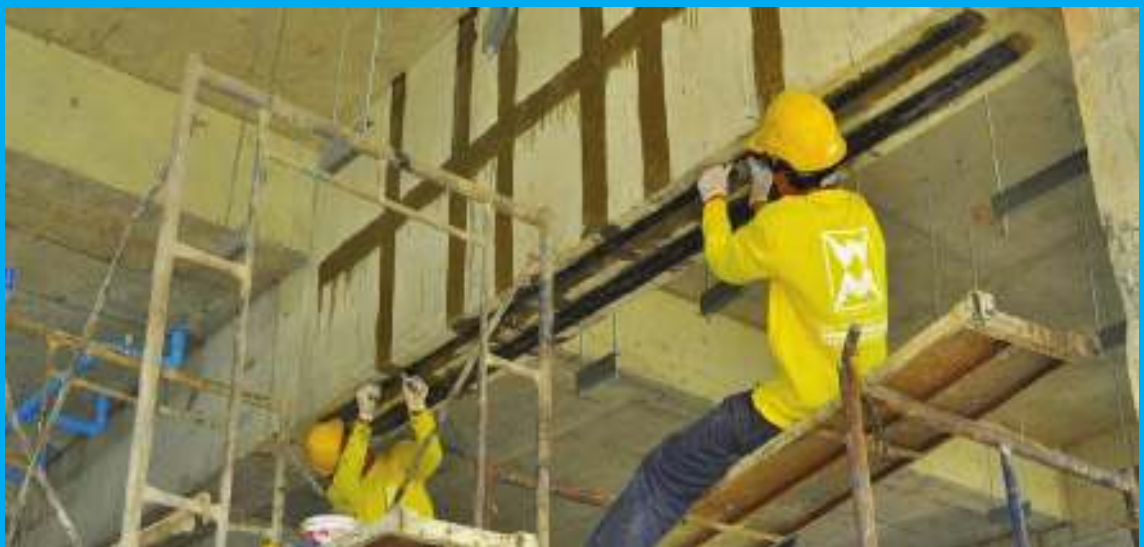
Carbon fiber strip strengthening to concrete beam
